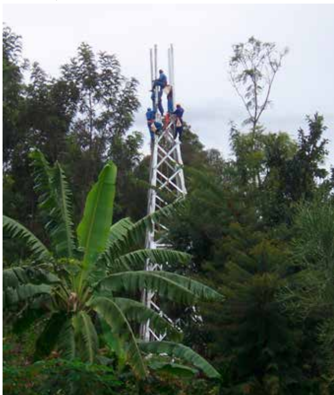
Construction of a transmission tower
