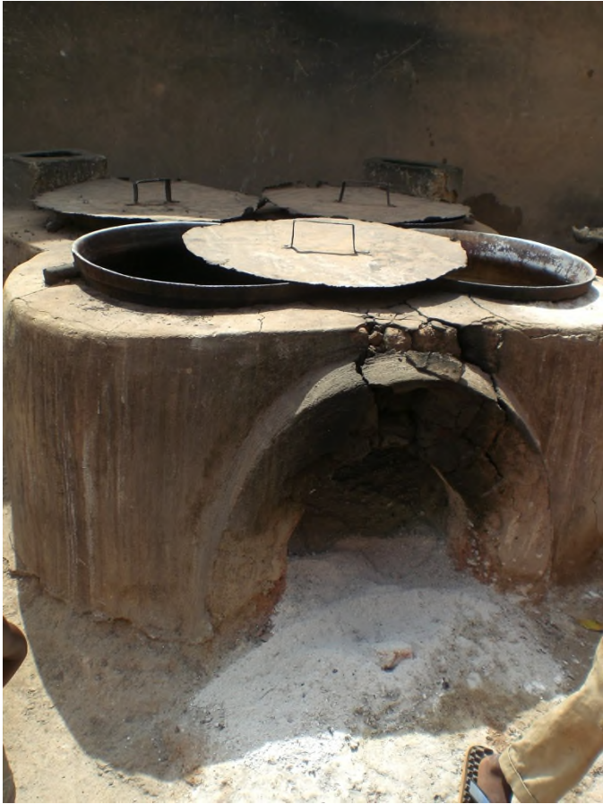
Photo 8: A Roundé stove with a broken door (a)
