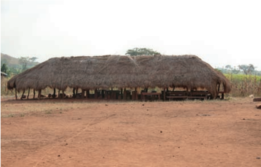
Temporary classroom of the rural St. Livingstone primary school, Masindi.
