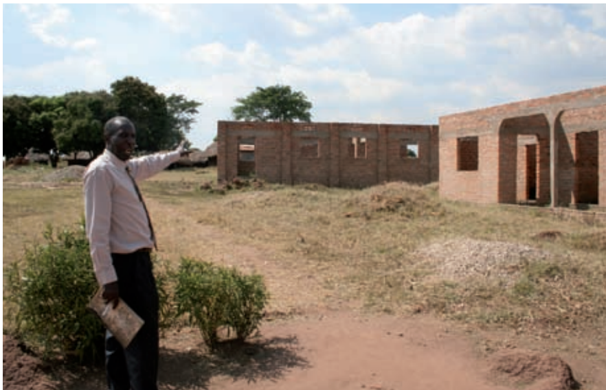
Construction of new classrooms at Kiryandongo BCS, Masindi.
