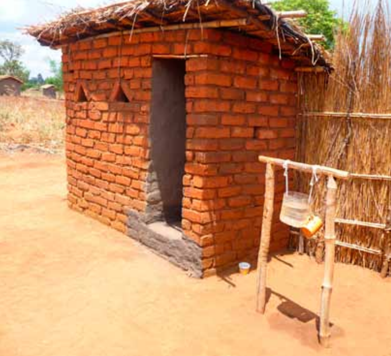
Latrine with handwashing facility
