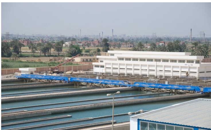
Photo: Construction of a water treatment plant Egypt (IOB, 2011)
