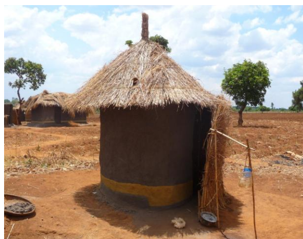
Photo: A basic latrine in Mozambique (IOB, 2011)
