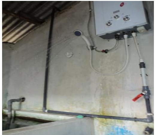
A water heater running with biogas
