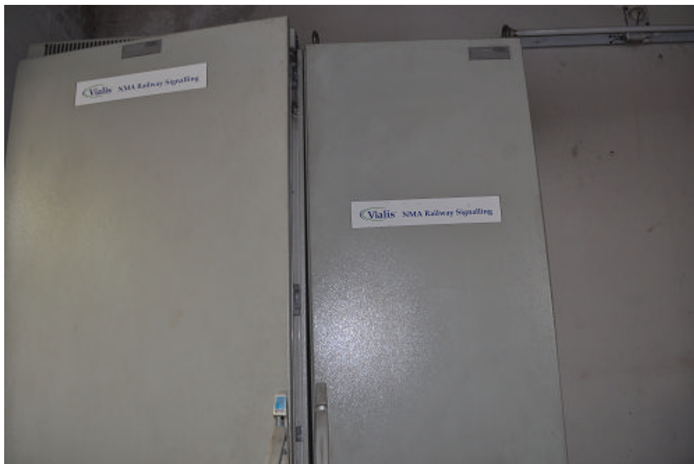
Photo 2: Installed Vialis Equipment (1)
