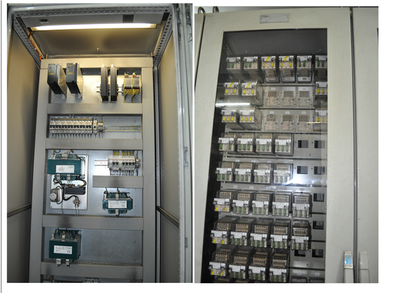
Photo 3: Installed Vialis Equipment (2)
