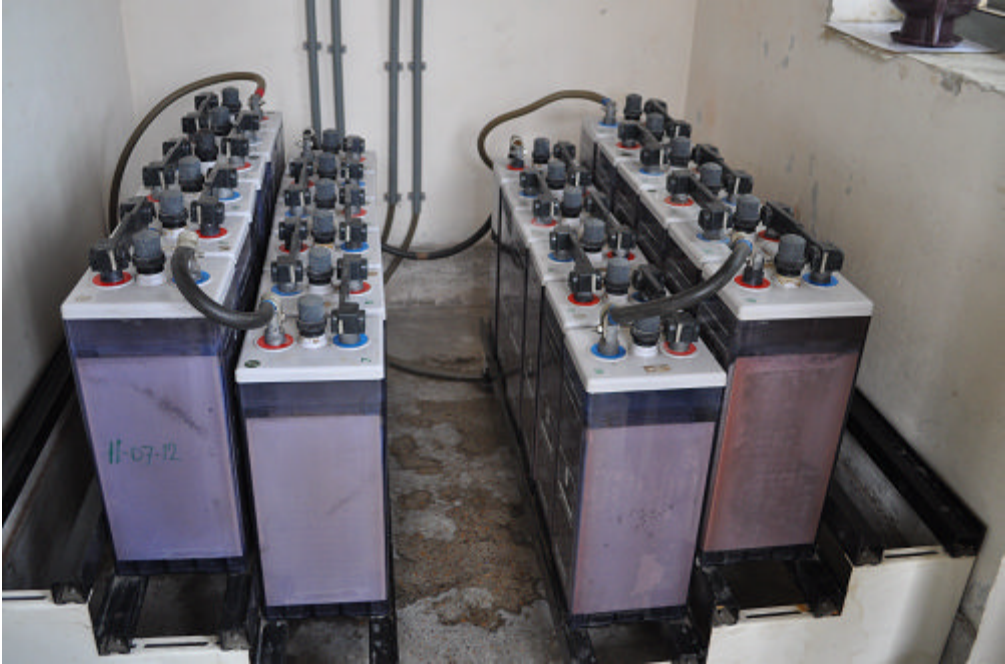
Photo 4: Complementary Equipment: Batteries and a Generator
