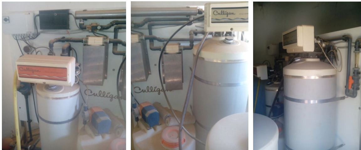
Photo 1: Water Softeners at Manyoni District Hospital, 2014
